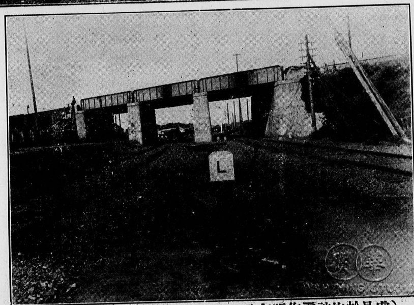
被日軍折毀之京奉路線(在一九二八年張作霖被炸於是處) One of the rails of the Peking-Mukden line torn up by the Japanese. This is the very place where Marshal Chang Tso Lin was bombed to death by order of Tanaka as is supposed by many.
